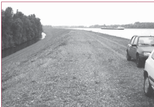
▲ Figure 10 – Digue rase.
