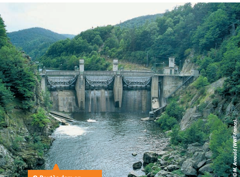
④ Poutès dam on the upper Allier river.
