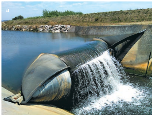
2 View of the irrigation district: a) inflatable weir (to supply sector C7); b) main lined canal (sector C2B); c) secondary canal and surface irrigated field (sector C7); d) maize furrows irrigation with distribution by siphons from a earth canal (sector C5); e) field irrigated by traveller-gun sprinkler irrigation (sector C1A); f) pepper field drip irrigated (sector C1B).
